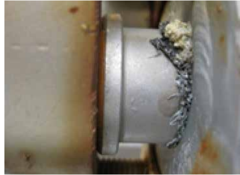
Figure 2: Improper installation: packing out stuffing box
