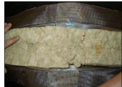
6. Butt Insulation Over Splice
