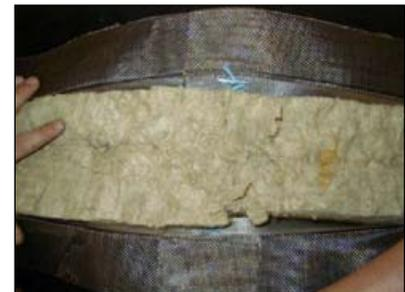
6. Butt Insulation Over Splice
